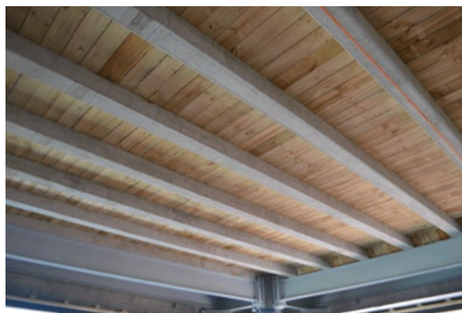
Figure 2 - Example of rib and timber infill flooring systems
