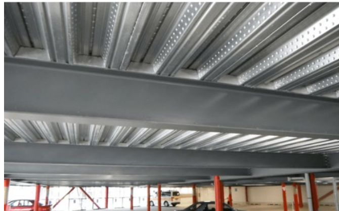
Figure 1 - Example of composite concrete flooring systems
