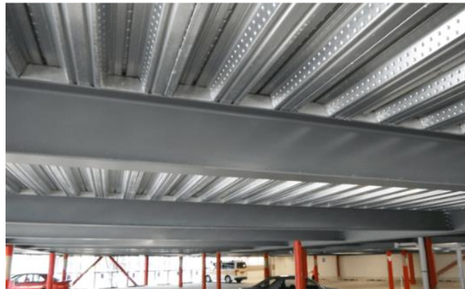
Figure 1 - Example of composite concrete flooring systems
