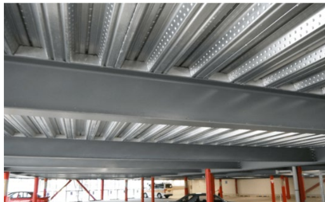
Figure 2 - Example of composite concrete flooring systems
