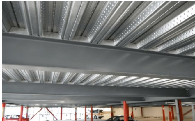
Figure 2 - Example of composite concrete flooring systems
